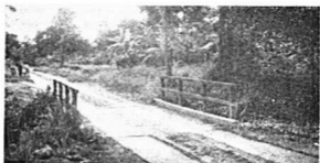
A kampong road with a new bridge provides access to secluded kampongs in the district of Gelang Patah in Johore.
